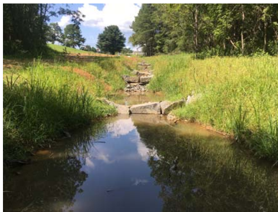
Figure 2: Step pools in restored stream allow water to slow and pollutants to filter out. Photo credit: Ecosystem Services
